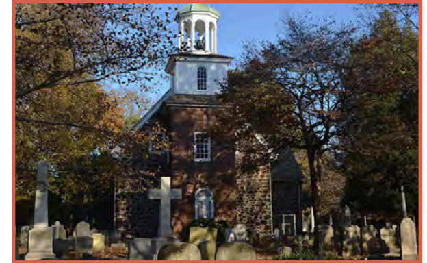
Old Swede's Church. Source: Old Swede's
