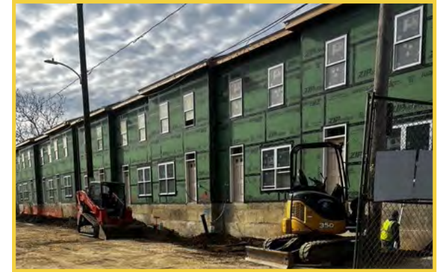
New construction in the Eastside. Source: Habitat for Humanity
